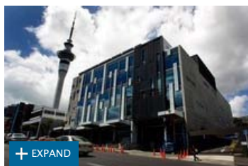
Manson TCLM at 162 Victoria Street in central Auckland is almost completed. Photo / Sarah Ivey
